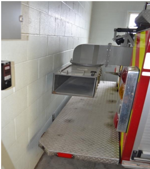
Figure 14. Proximity of the fire apparatus to the bay wall.
