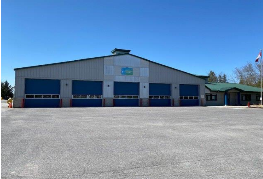
Figure 11. Exterior of Station 1 (Almonte).
