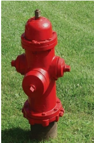
Figure 9. Example of a private hydrant.
