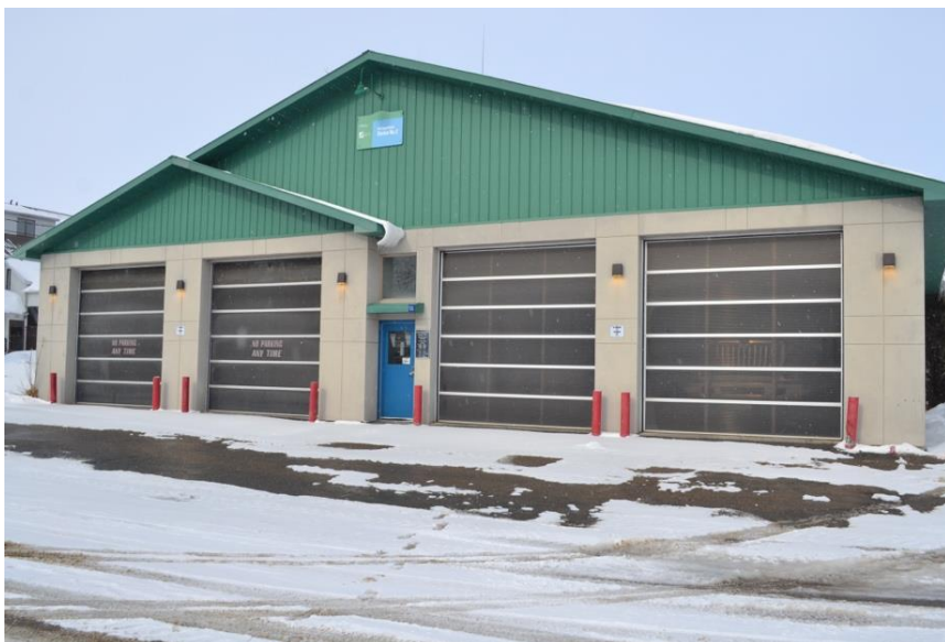
Figure 12. Exterior of Station 2 (Pakenham).
