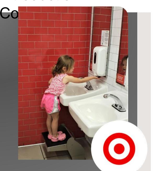
There is a product called the "Step 'n Wash" that can help. The Step 'n Wash is simple but very effective. It is a self-retracting step that installs under the sink counter in public washrooms. You simply push it down with your foot and it provides a step so you can stand high enough to wash your hands without getting your sleeves or shirt wet.
