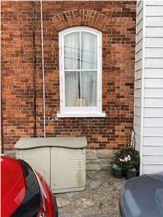
Photo 2. Back Elevation – A close up of window to be replaced.
